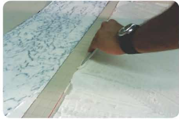
Back Fill and Trowel
